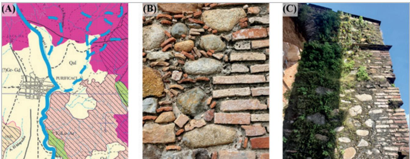
**Figure 7-** (A) Pluvial causes. (B) Rounded-edged stones on the second buttress in front of the gate. (C) First buttress behind the tower, damage mainly to bricks and mortar.
